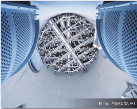
PP-H blast lances and strainer baskets in the flue-gas desulphurisation system of a coal-fired power plant
