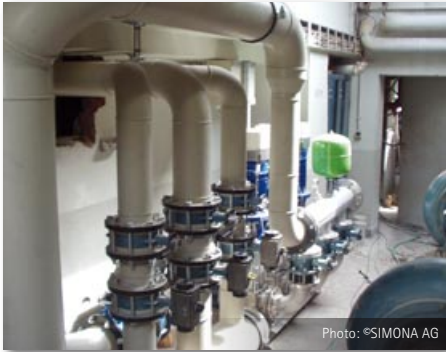
Distribution system showing PP-H piping and fittings in a water-preparation plant
