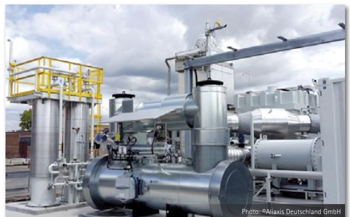
1.4 Megawatt fuel cell (MCFC) supplying energy to the production location
