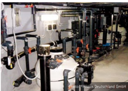
Desalination plant showing PE100 pipes and fittings
